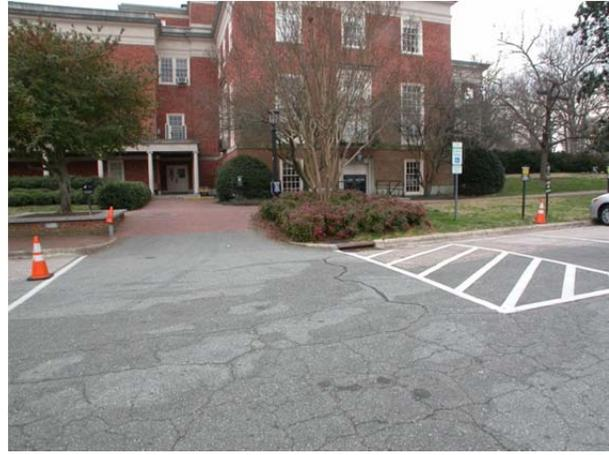
**Figure 3 – Inaccessible Western Curb Ramp**
