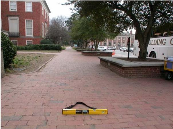
**Figure 4 - 7.6% Cross Slope on Approach Walk**
