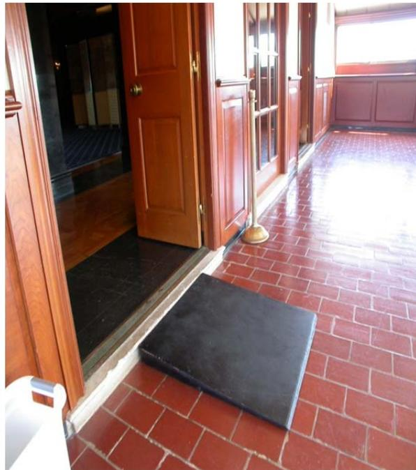
**Figure 9 - 9.7% Portable Wood Ramp**
