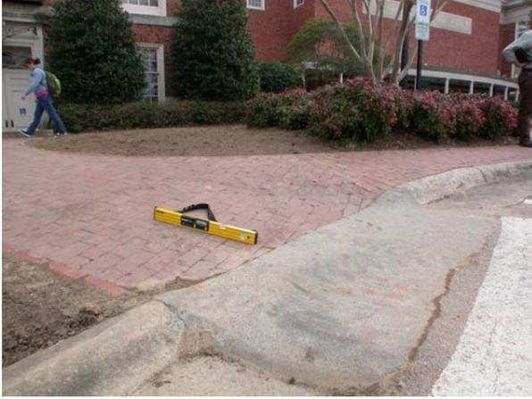
**Figure 2 – Inaccessible Eastern Curb Ramp**
