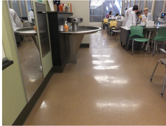
Figure 11. Hand Sink not Cane Detectable
