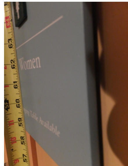
Figure 16. No Tactile Signage
