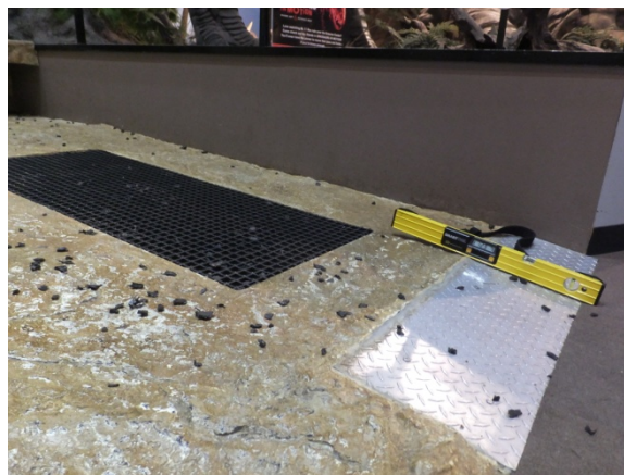
Figure 12. Ramp with 12.9% Slope
