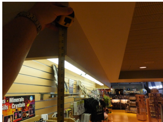
Figure 8. Low Soffit in Explore Store
