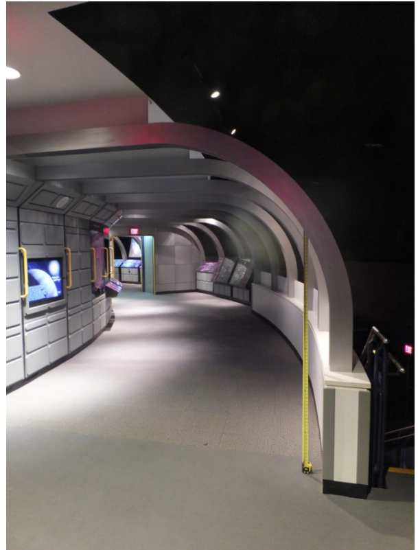
Figure 27. Less than 80" Height at Curved Structure
