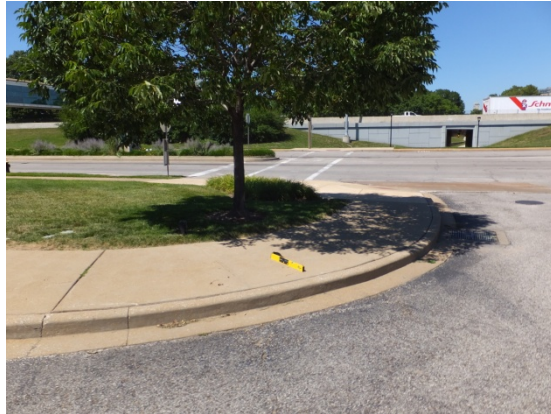
Figure 5. Approach with 5.4% Cross-Slope
