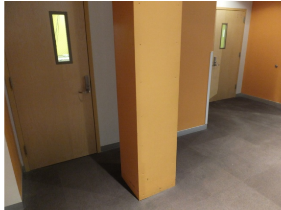
Figure 14. Column Blocks Meeting Room Door
