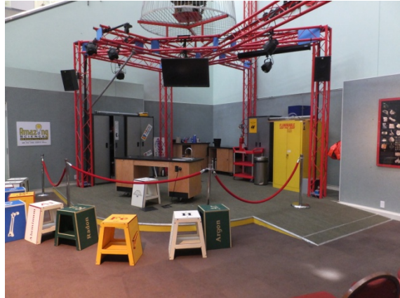
Figure 13. Stage Ramp Lacks Edge Protection
